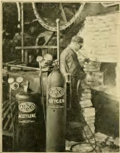
Fig. 125. — Welding with an acetylene torch. A cracked cylinder of a locomotive is being welded just inside the opening in the temporary brick wall
