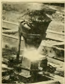
Fig. 180. — Welding a steel rail with thermit. Sketch of the crucible and mold in position (right). The operation is shown on the left
