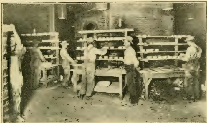
Fig. 192. — Scene in the largest chemical porcelain works in the United States. Putting porcelain dishes in clay boxes preparatory to heating in the kiln
