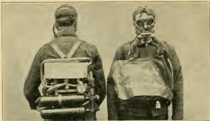
Fig. 11. — Man equipped with oxygen-breathing apparatus. He breathes through his mouth from the gas bag carried on his chest ( right ). The tank of oxygen and the regenerating can are carried on his back ( left )
