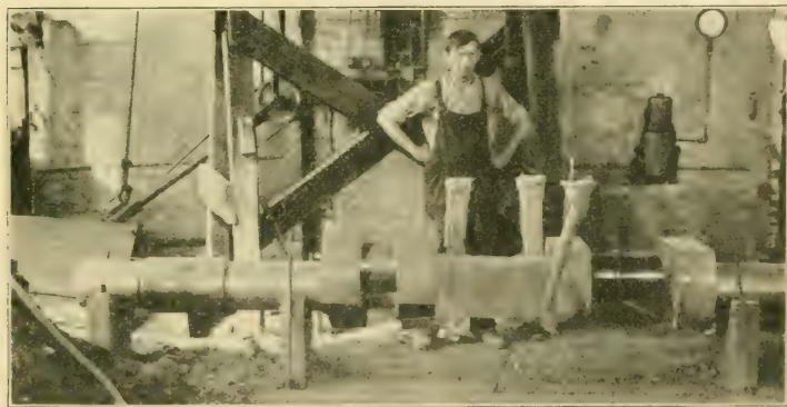
Fig. 190. — A crankshaft repaired by the thermit process
