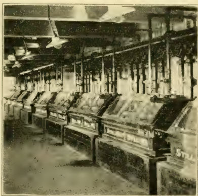
Fig. 113. — Look boxes in which the distillates can be examined as they flow from the condensers through the receiving house on to the special storage tanks
