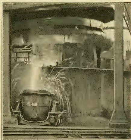
Fig. 173 — Tapping a blast furnace
